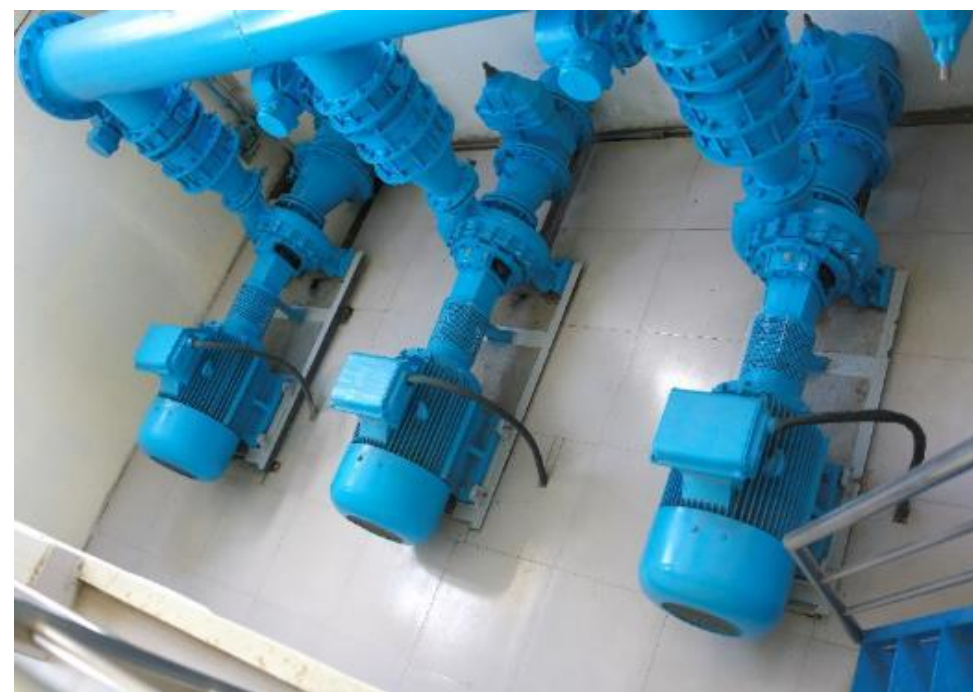
Tu Ha WTP Water distribution pump (Existing pump)
