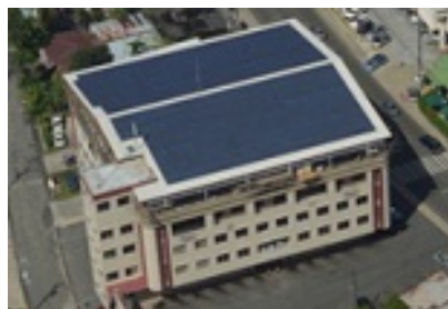
Rooftop solar PV AEON Mall, Pacific Consultants, Asian Gateway Corp., etc.
