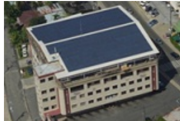
Installing solar PV system, PCKK, Palau, Maldives
