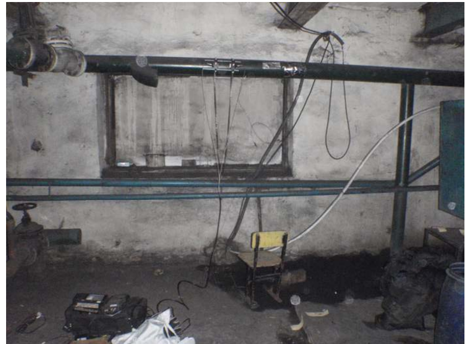
Reference Boiler at 87 school
