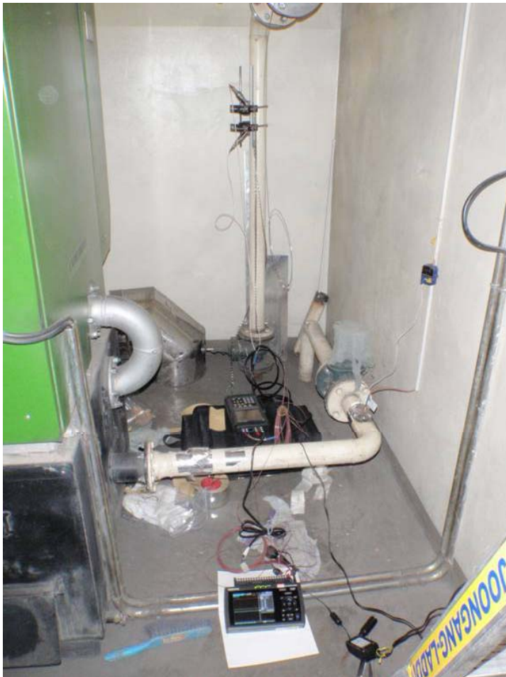
Project Boiler at 79 school
