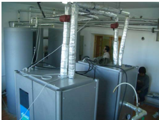
Heat pumps and storage tanks at school
