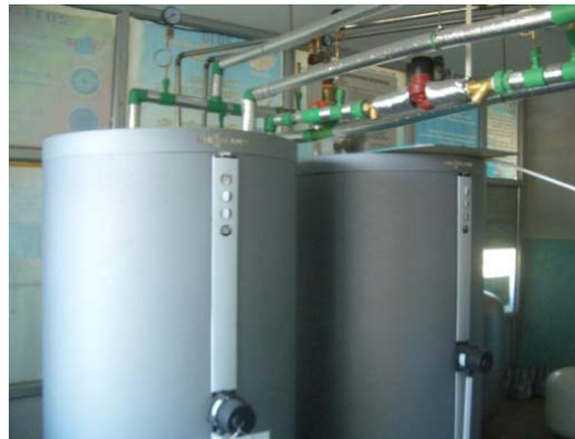
Storage tanks at kindergarten
