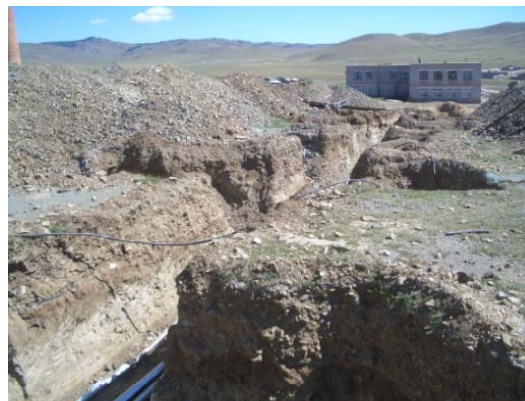
Underground geo-thermal piping at school under construction
