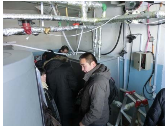
On-site investigation at the kindergarten
