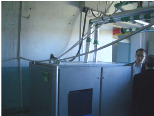
Heat pump at kindergarten
