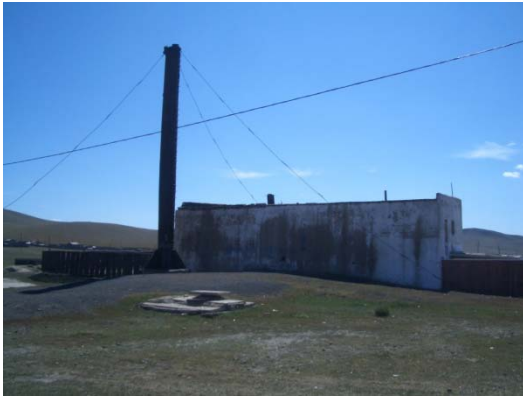
Boiler plant in Zuumod
