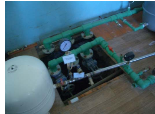
Geo-thermal piping at kindergarten
