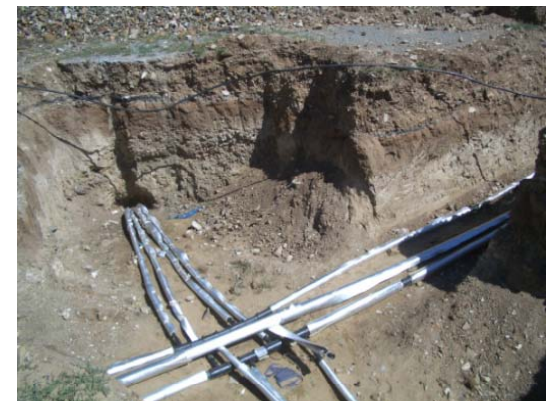
Underground geo-thermal piping at school under construction
