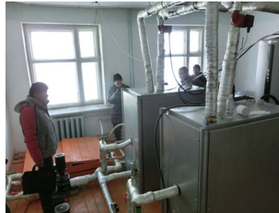
On-site investigation at the school
