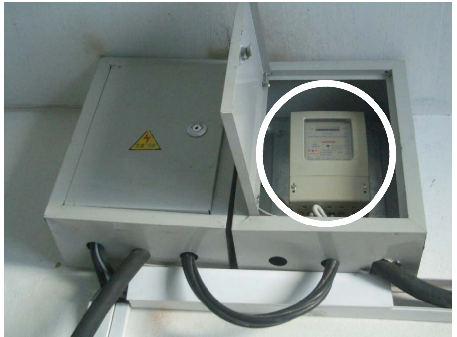
Watt hour meter at kindergarten
