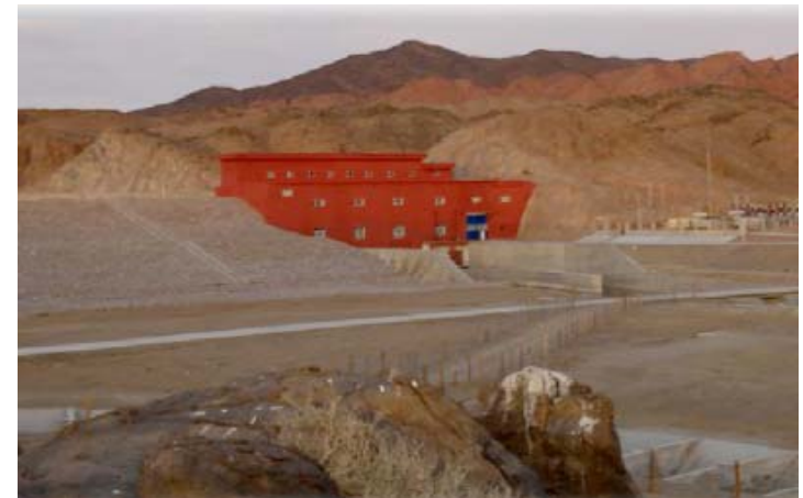
Durgun Hydro Power Plant
