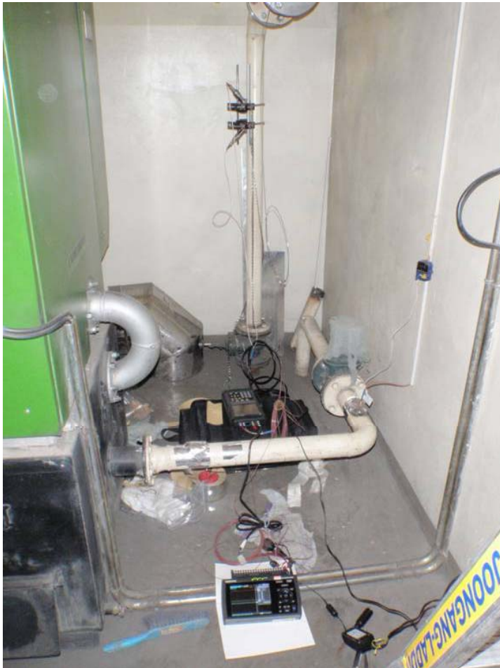
Project Boiler at 79 school
