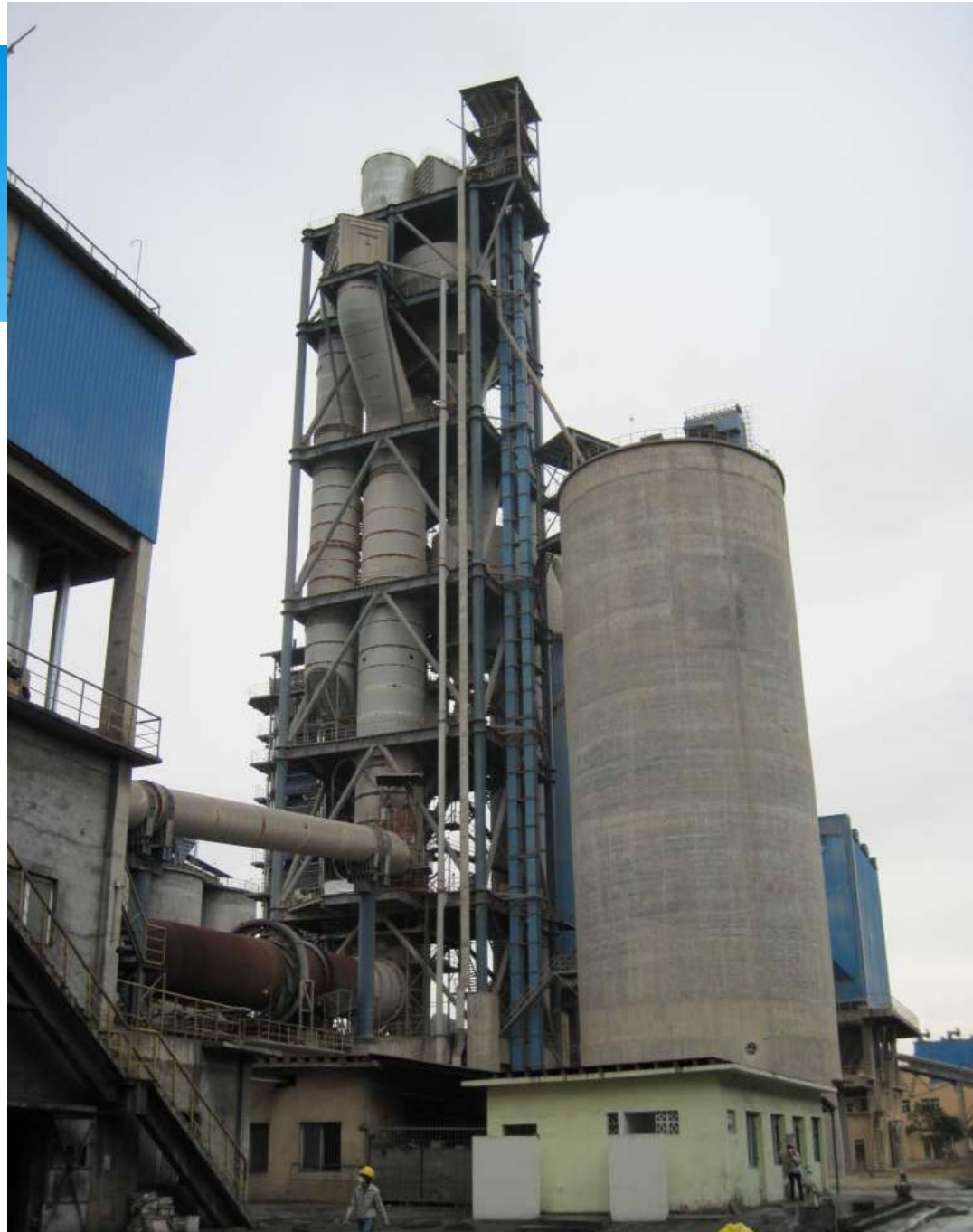
Example of dry process plant (similar to project capacity)
