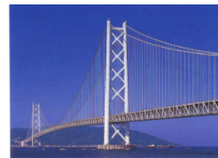
Akashi-Kaikyo Ohashi Bridge
