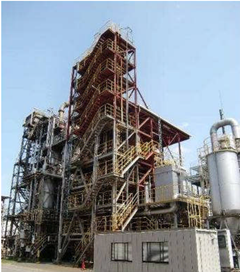
CFB PILOT TEST FACILITY OVERVIEW
