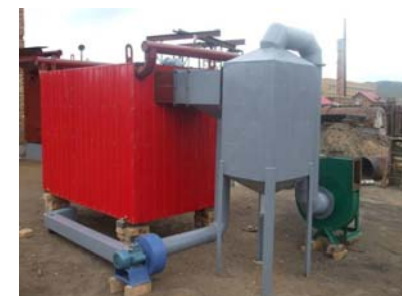
High-efficiency heat only boiler
