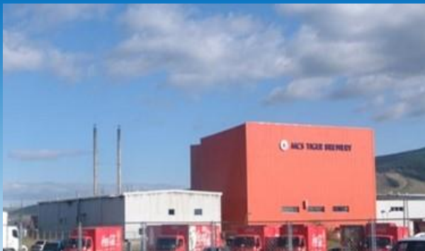
Introduction of Heat Pumps or Thermal Storage Heater
