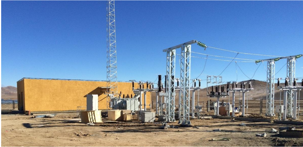
35/10kV Monnararan substation
