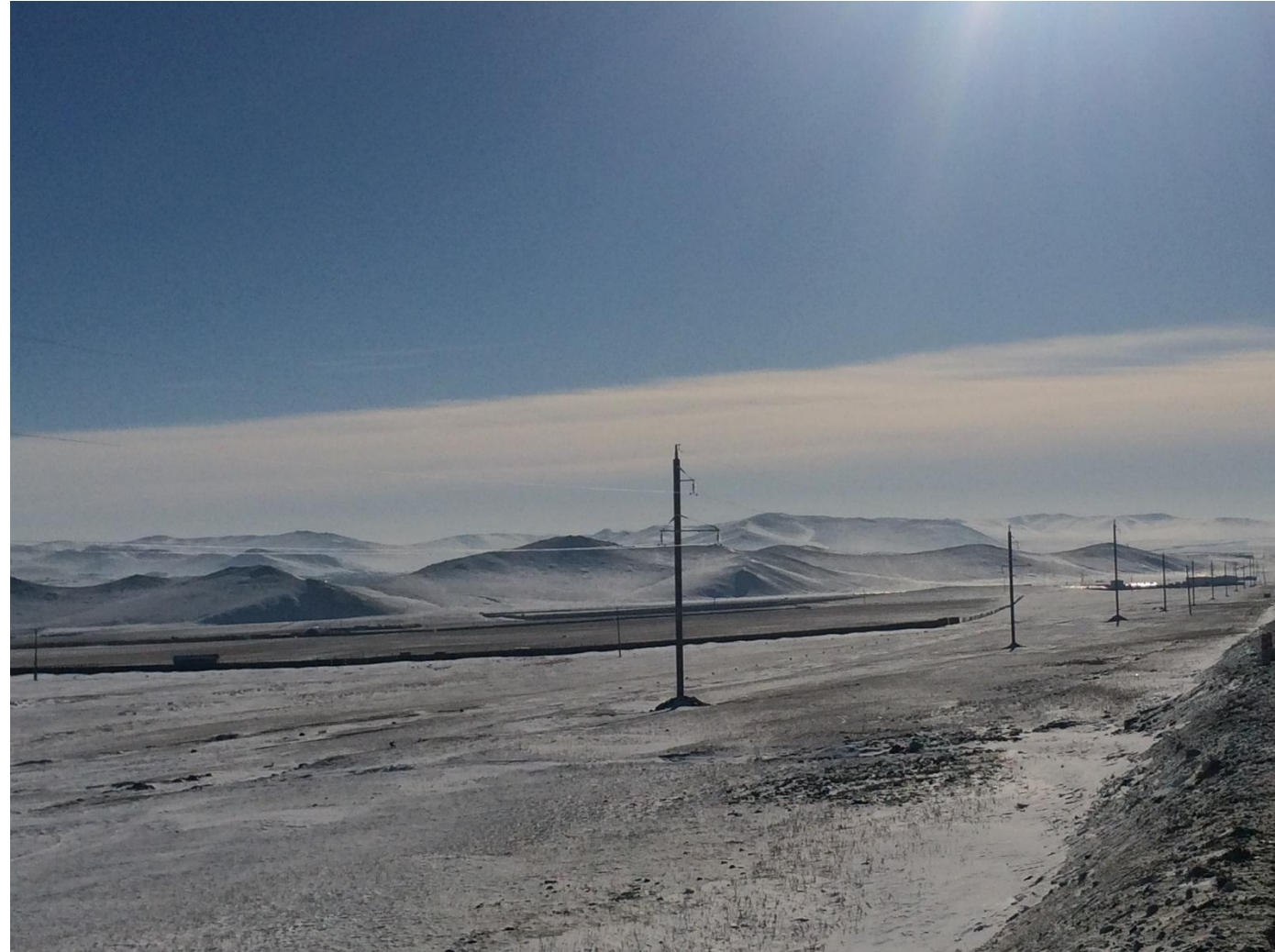
35kV Transmission line
