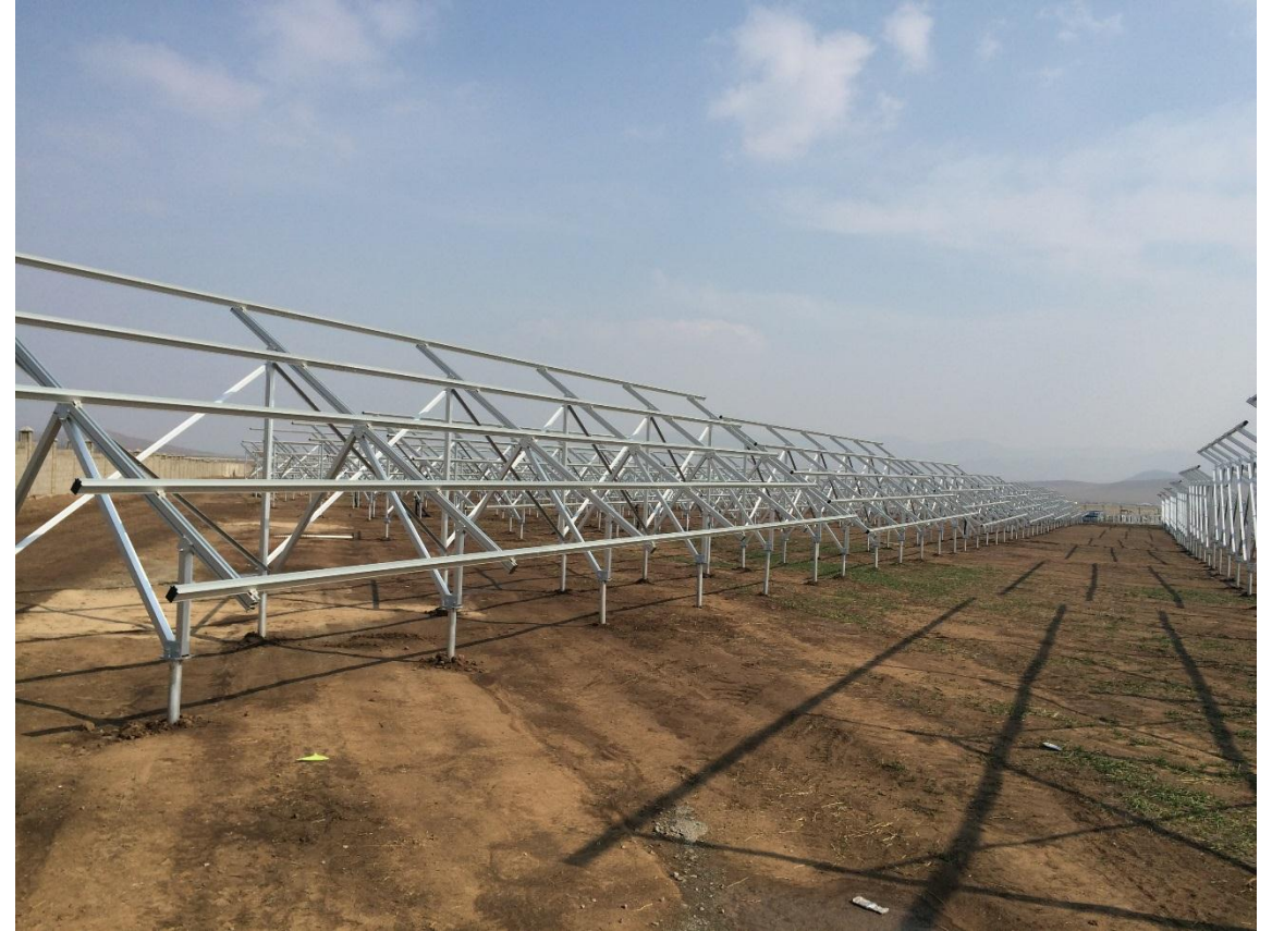
Assembling the PV module mounting frames
