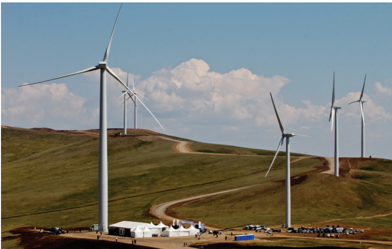
Figure 1-4: 50 MW Salkhit wind farm, Mongolia
