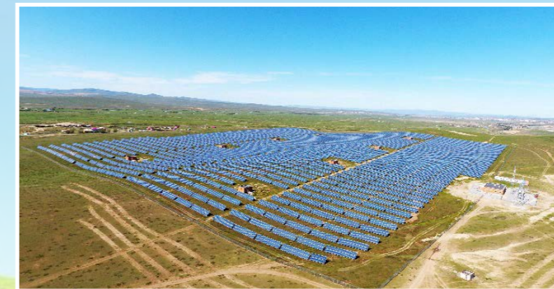
10MW Solar Power Project in Darkhan City
