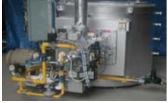
Regenerative Burners in industries, Toyotsu Machinery, Indonesia
