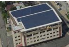
Installing solar PV system, PCKK, Palau Maldives
