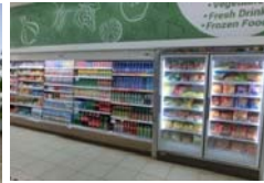
Energy saving at convenience stores, Panasonic, Indonesia
