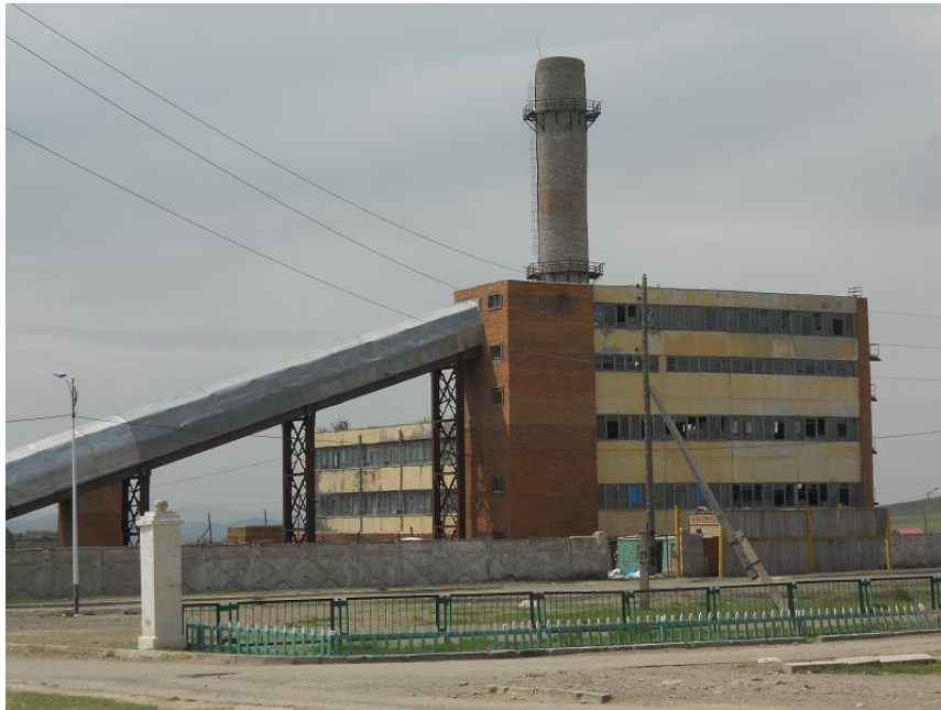
A local Heat Only Boiler (HOB) in Tuv Aimag, Mongolia
