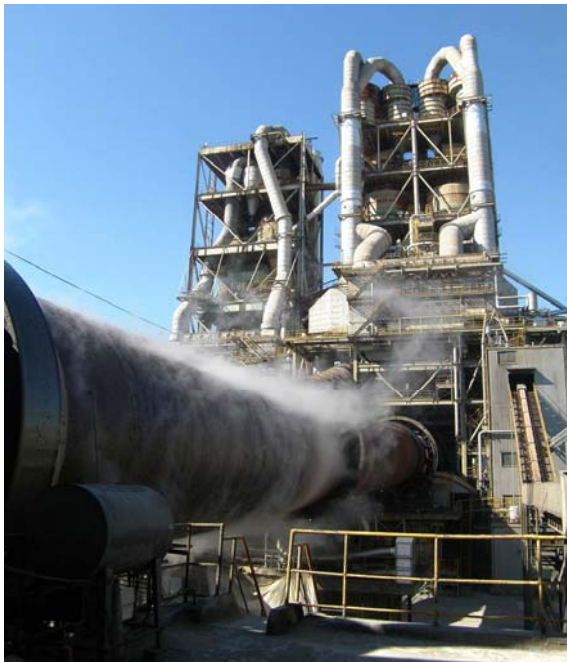
Preheater (back) of 65m in height and Rotary kiln (fore) of 5.4m in diameter, 95m in length, 3200 ton/day production capacity, 250 kW powered
