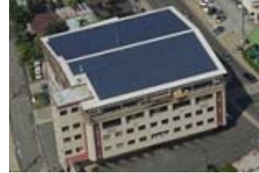
Installing solar PV system, PCKK, Palau Maldives
