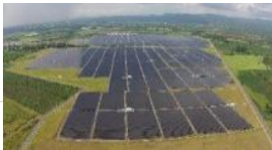
83MW NED Plant in Thailand
