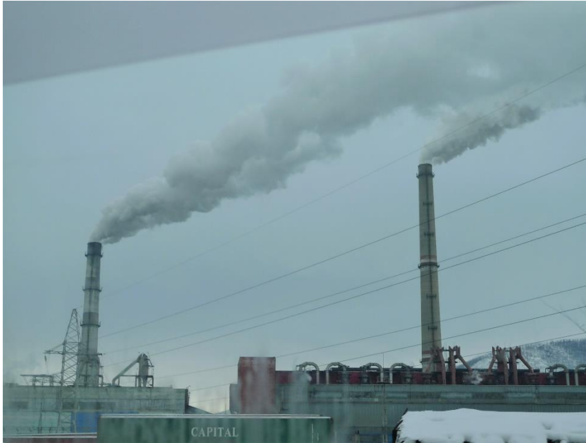
Gas emission by coal fired heat and power plant at Ulaanbaatar
