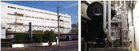
Tokyo Toyomi Cold Storage Funabashi Logistic center
