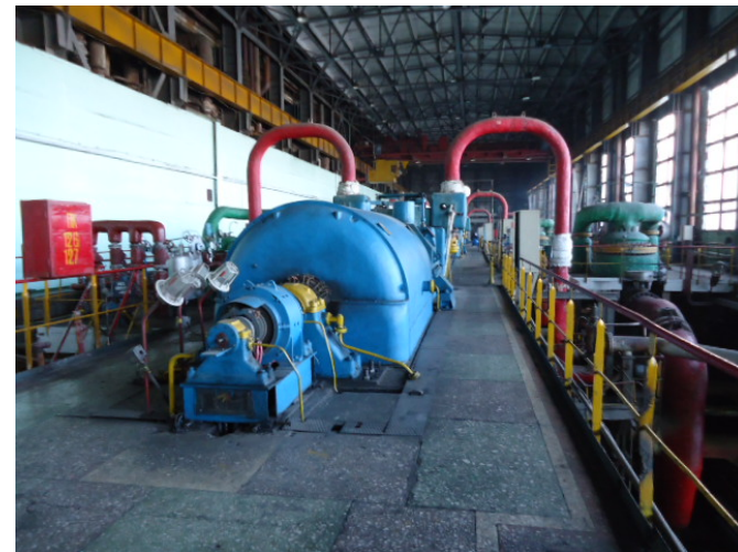
Turbine in CHP3
